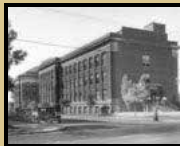
Zoology Building, constructed 1915
